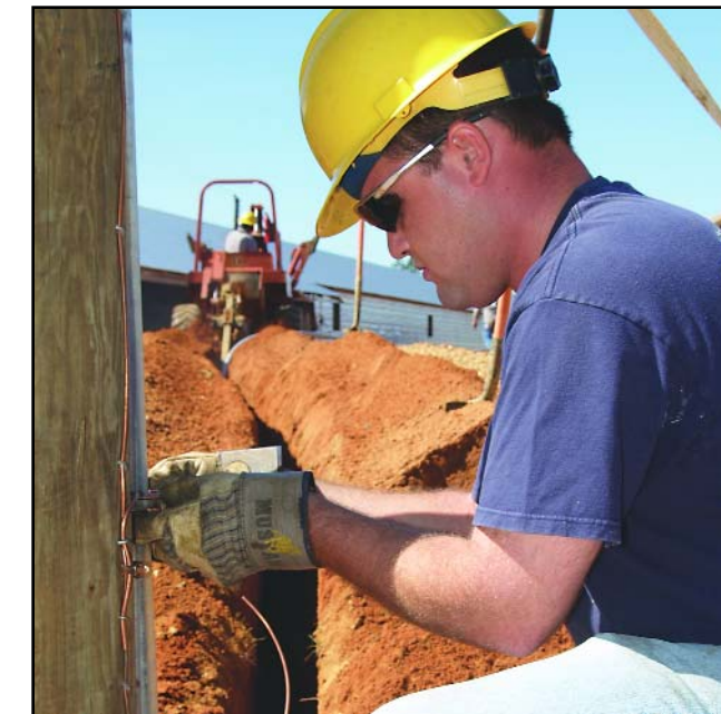
Southern Pine's Brandon district underground crew (left) builds service to a new subdivision home in Rankin County. The Taylorsville district underground crew (above) buries lines to serve new poultry houses in Smith County.
